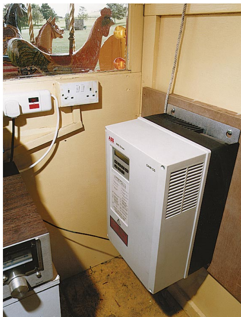
Remote panels allow the frequency converter to be installed in the security of a central service cubicle.
