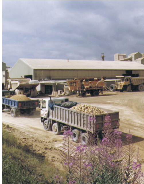
Redland has installed an a.c. drive, supplied by Slater Drive Systems, at its Thrislington aggregate plant.
