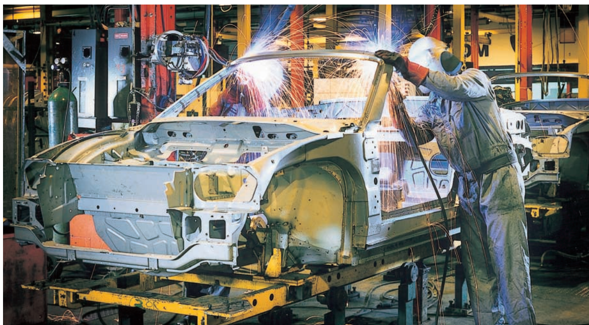
Over 85% saving in the running cost of paint plant motors is being achieved by Coventry-based vehicle body panel manufacturer, Mayflower Vehicle Systems, following the installation of ABB AC drives by ABB Drives Alliance Partner Sentrige Control
