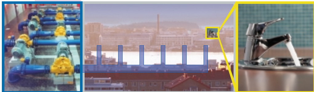
Figure 1. In domestic buildings, the fresh water pump's variable output flow is controlled according to water consumption, which is low at night but high in the mornings and evenings. If you are showering, it is important that water flow and temperature are constant. As a result, disturbances such as water pressure variation must be countered by an effective process control.
